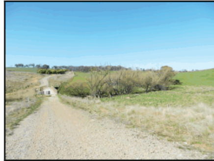
Above: Crossing on the Carcoar-Millthorpe Road at the Cowriga Creek - site of the new bridge. Photo" G. Stanbridge
